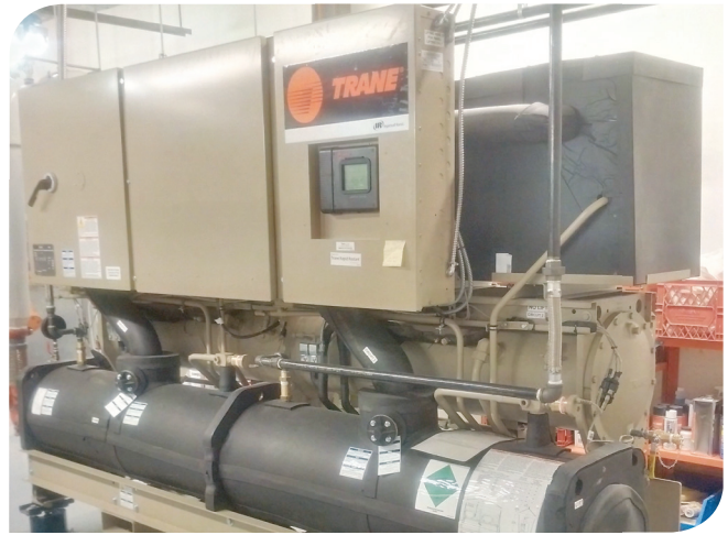
Trane® Series R™ Helical Rotary heat reclaim chiller provides the Vancity Centre building with reliable, energy efficient operation.
